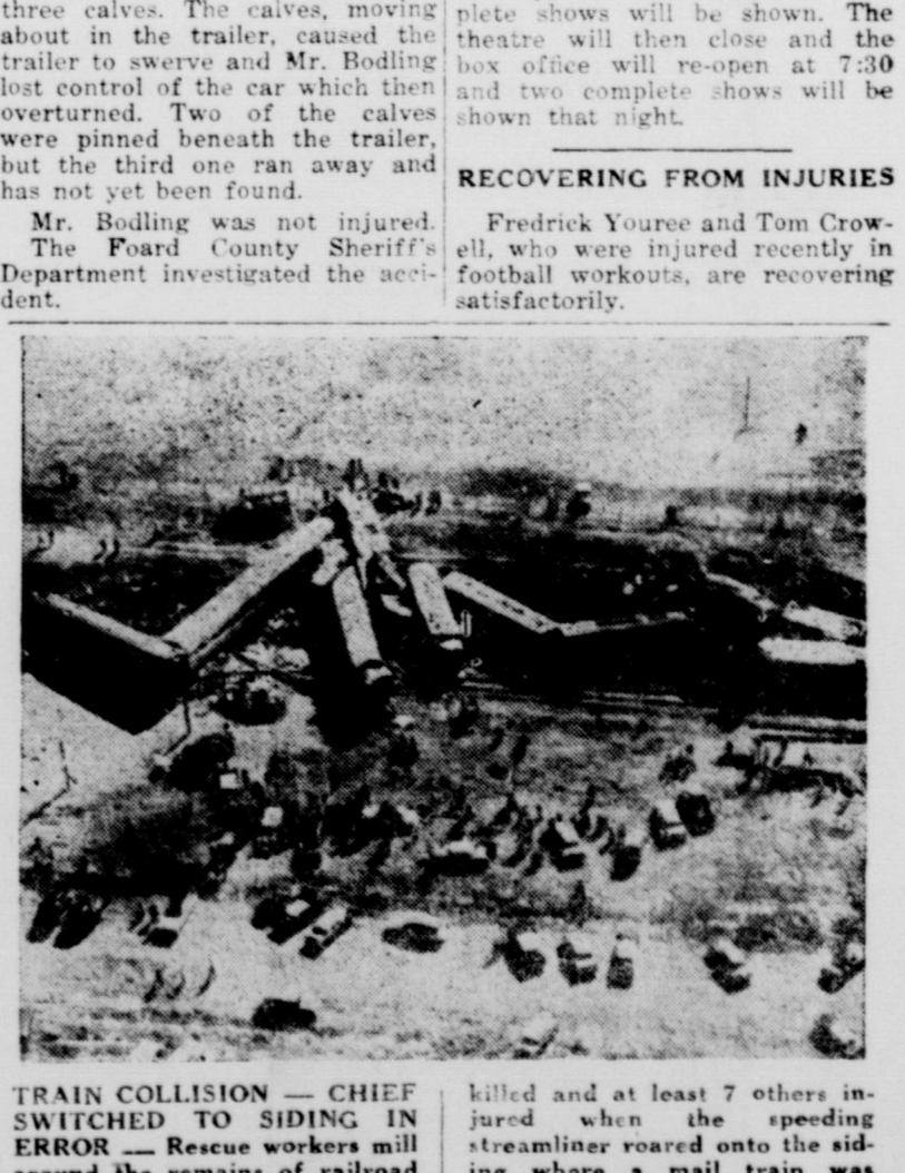
TRAIN COLLISION — CHIEF SWITCHED TO SIDING IN ERROR — Rescue workers mill around the remains of railroad cars of the Santa Fe Chief and a mail train near Springer, N. M. Twenty crew members were killed and at least 7 others injured when the speeding streamliner roared onto the siding where a mail train was waiting for it to pass. A switch was thrown in error by a yard worker.
