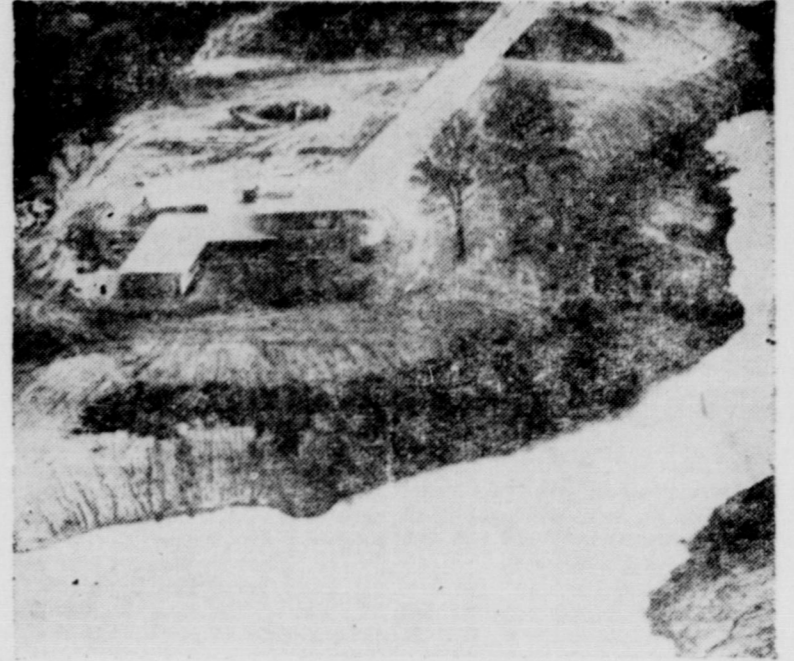
MAN-MADE ISLAND — Aerial view of man-made island reportedly being built as hangout for East St. Louis gang of hoodlum Frank "Buster" Wortman in the Bethel School area near Collins-
