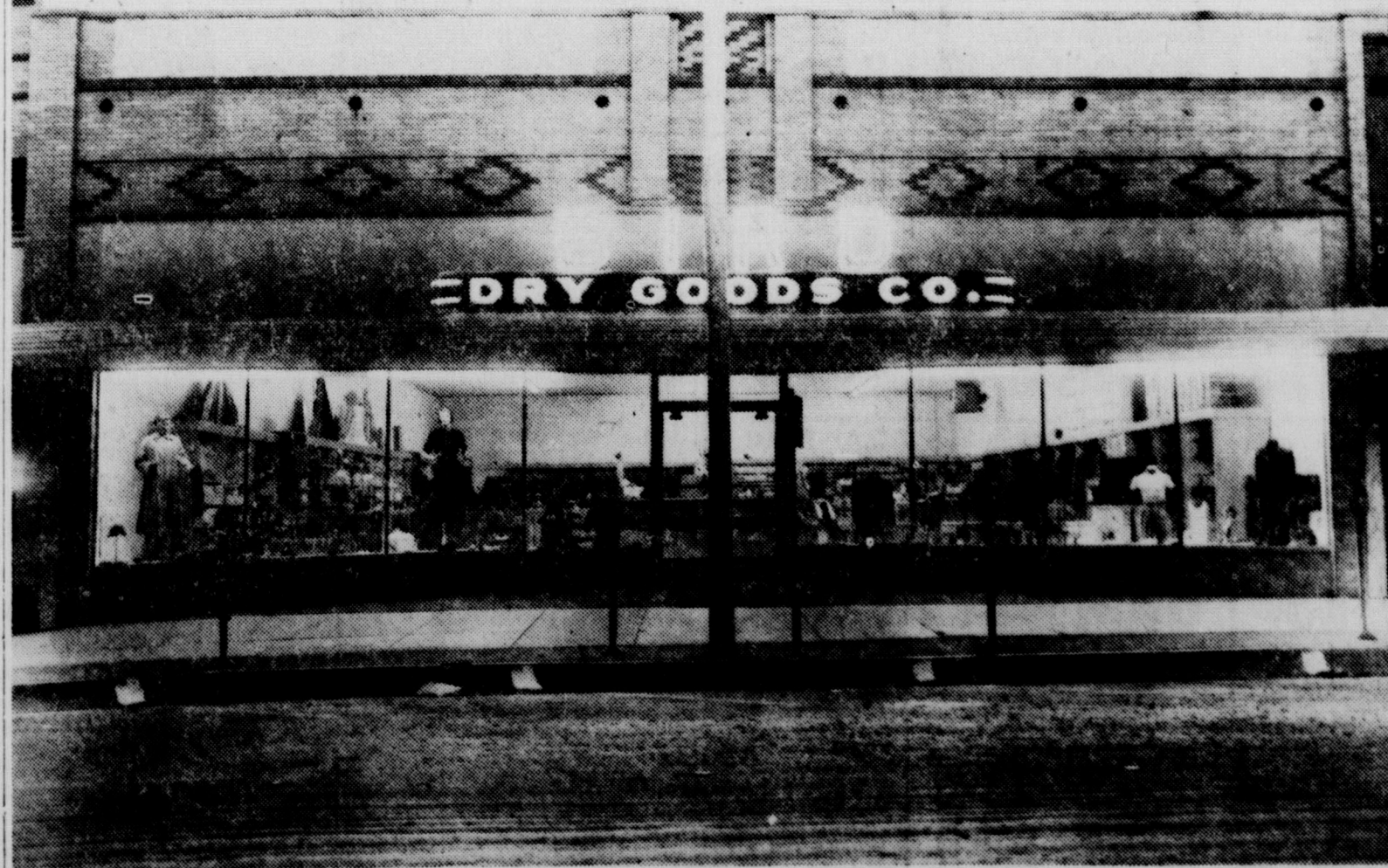
NEW HOME OF BIRD DRY GOODS CO.—Pictured above is the completely new and modern home of the Bird Dry Goods Company. The new business is located on the west side of the square in the same location as the Lanier building, which was destroyed by fire last December. Formal opening of this new business will be held tomorrow morning. (Photo by Robertson).
