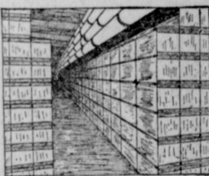
Egg Room in a Large Eastern Cold-Storage Plant.
