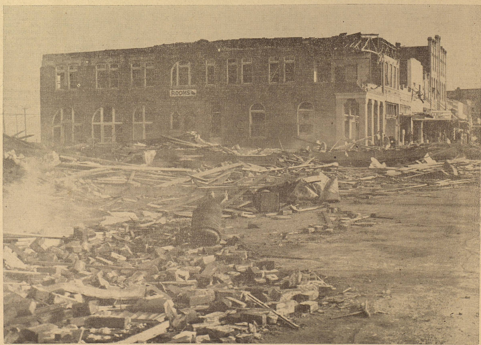
The main streets of Crowell were littered with bricks and debris Wednesday morning. In the scene above, looking north from the southwest corner of the square, the building seemed to have exploded with terrific force.
