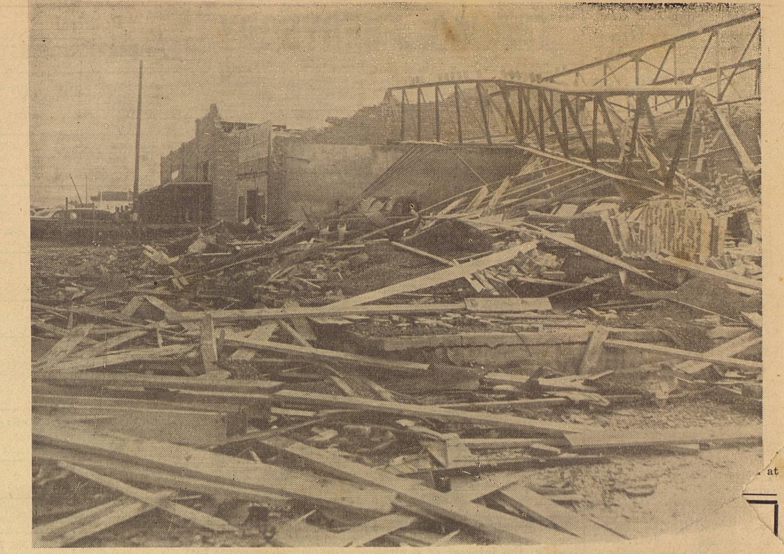
Damage to the east side of the square at Crowell is shown in the picture, made just as workers started clearing the wreckage. The Borchardt Chevrolet Company is shown in the foreground, with a number of new cars and trucks covered. Next in line is an auto supply store, The Foard County News, the first aid station and on the corner, a filling station that was converted into a cafe, supplied with food sent from neighboring towns. (Reporter-News Photo by Harry Holt)
