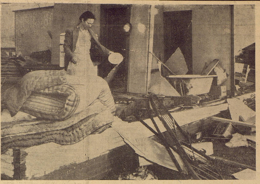
OPEN AIR HOME—Mrs. E. G. Anderson is pictured picking up the "remains" of household furnishings in her home in east part of Crowell. Directly back of Mrs. Anderson is a refrigerator that was not damaged and at right of the door there hangs a hat. (Reporter-News Photo)
