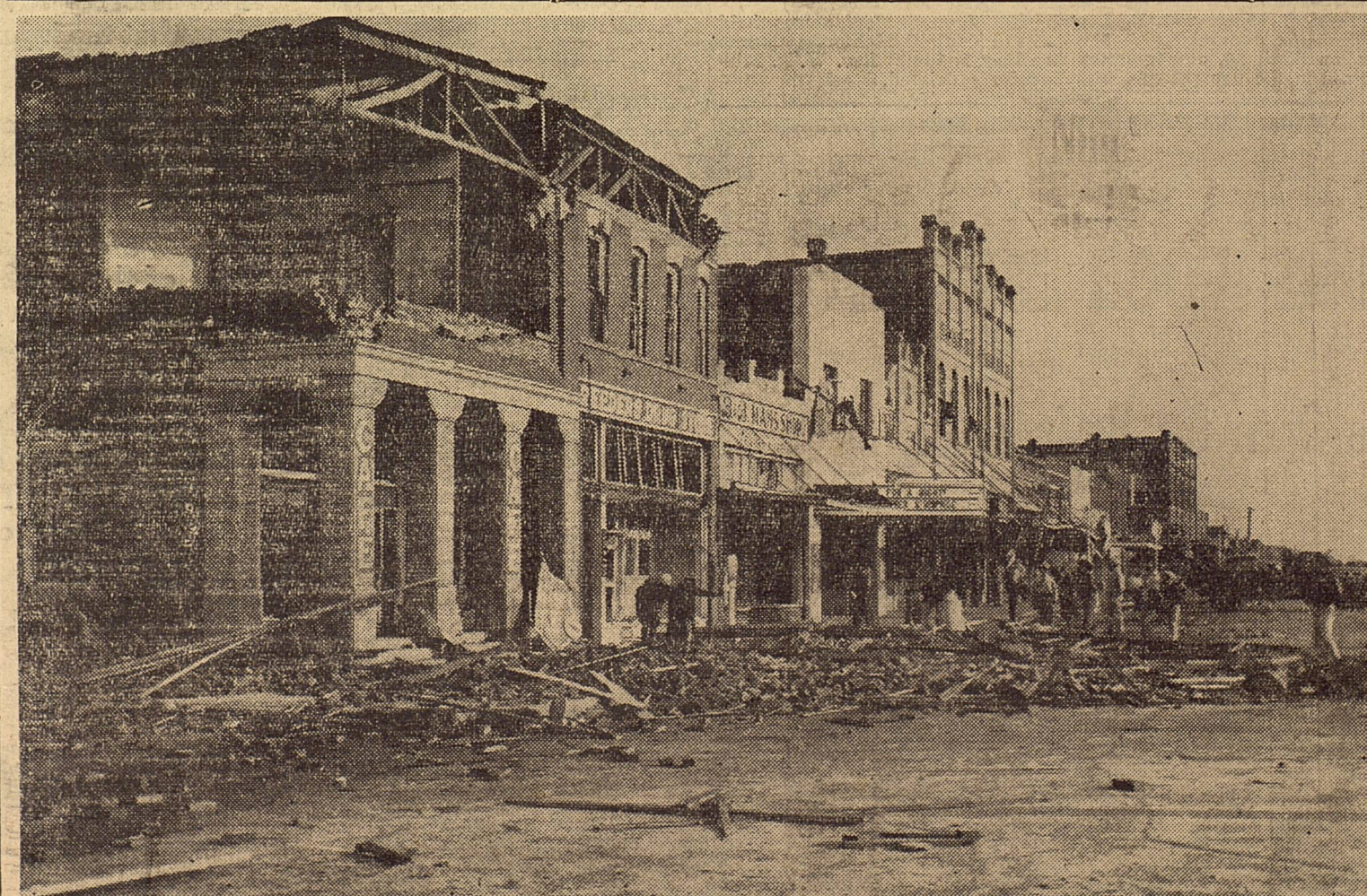
Looking north on the east side of the square at Crowell is the view of tornado damage. No business in this block escaped damage. Note that the highest structure, right center,
