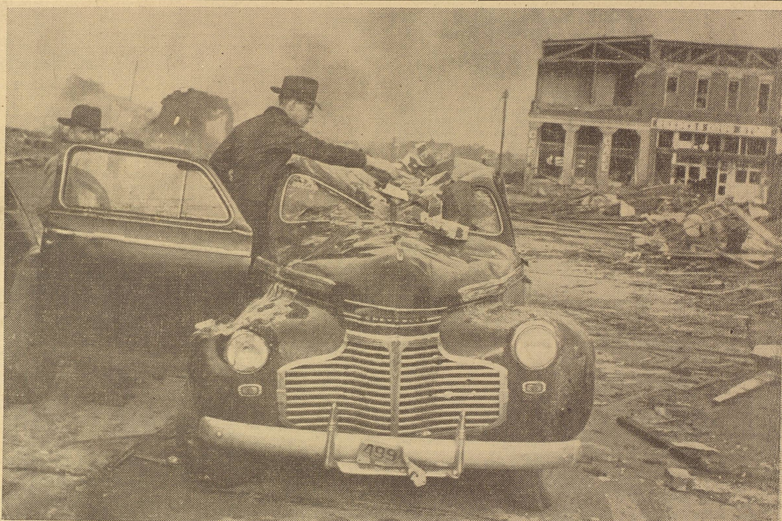
It rained bricks in Crowell Tuesday night for about 20 minutes and then hail stones almost as large as bricks fell, said Alfred Eddy, explaining the battered condition of his car. These bricks being removed apparently came from the top of the court house about 100 feet from the place where the car was parked.
