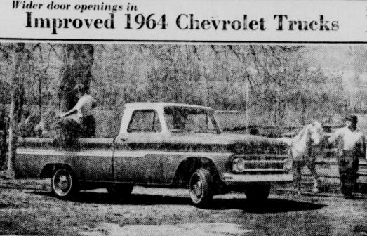
New forward slanting windshield pillar provides roomier door openings for easier entry and exit in 1964 Chevrolet trucks with regular cabs. Other features include longer lived lamps and exhaust systems, lower transmission hump in most pickup models, more positive door latches, and improved
