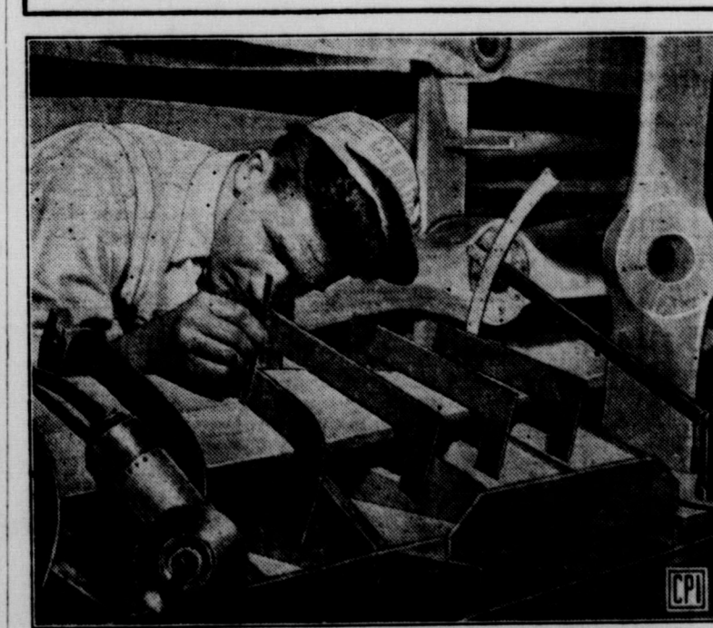
Passed by Censor THE manufacture of plane propellers from laminated wood requires the services of a keen eye and a steady pair of hands. Both blades must be identical in pitch to the merest fraction of an inch and the care exercised in measuring the pitch is indicated in the illustration. Laminated wood propellers have several advantages over those made of metal. They are lighter; they cost less and when struck by bullets or shell fragments, they split instead of twisting. One of the largest propeller plants in Canada is located in Winnipeg. Before the war it produced propeller-driven snowmobiles which are used extensively for winter trucking in those sections of the north beyond the reach of highways or railroads.
