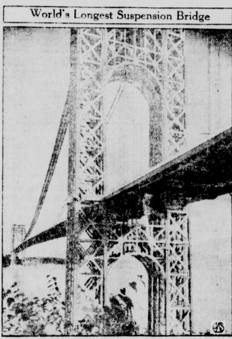
The George Washington Bridge across the Hudson River, opened on October 23, is two-thirds of a mile long between spans. It cost $60,000,000 and took four years to build. It is expected to pay for itself by tolls, after which it will be free to traffic between New York City and Northern New Jersey.
