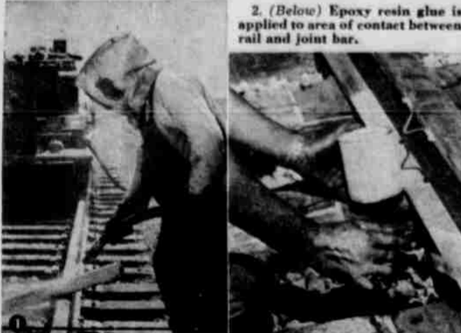
1. (Above) Joint bars and rail ends are sandblasted prior to application of epoxy glue.
