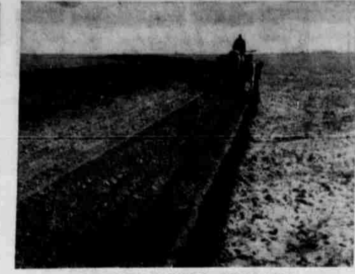
CONSTRUCTING TERRACE This Soil Conservation Service photo shows L. G. Thuett Jr. constructing a terrace with an elevator terracer on a Thuett farm west of Post.
