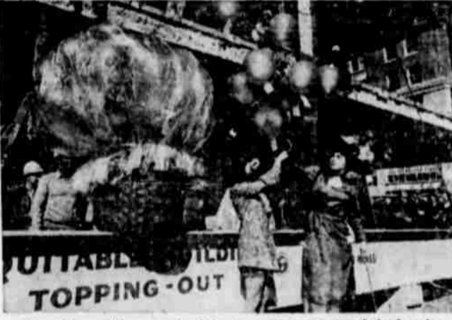
The old and the new in Atlanta were portrayed during festivities heralding "topping-out" of the 34-story steel framework for Equitable Life's new Southern headquarters building. Girls wear dress styles of today and 1892, when the company built Atlanta's first skyscraper.
