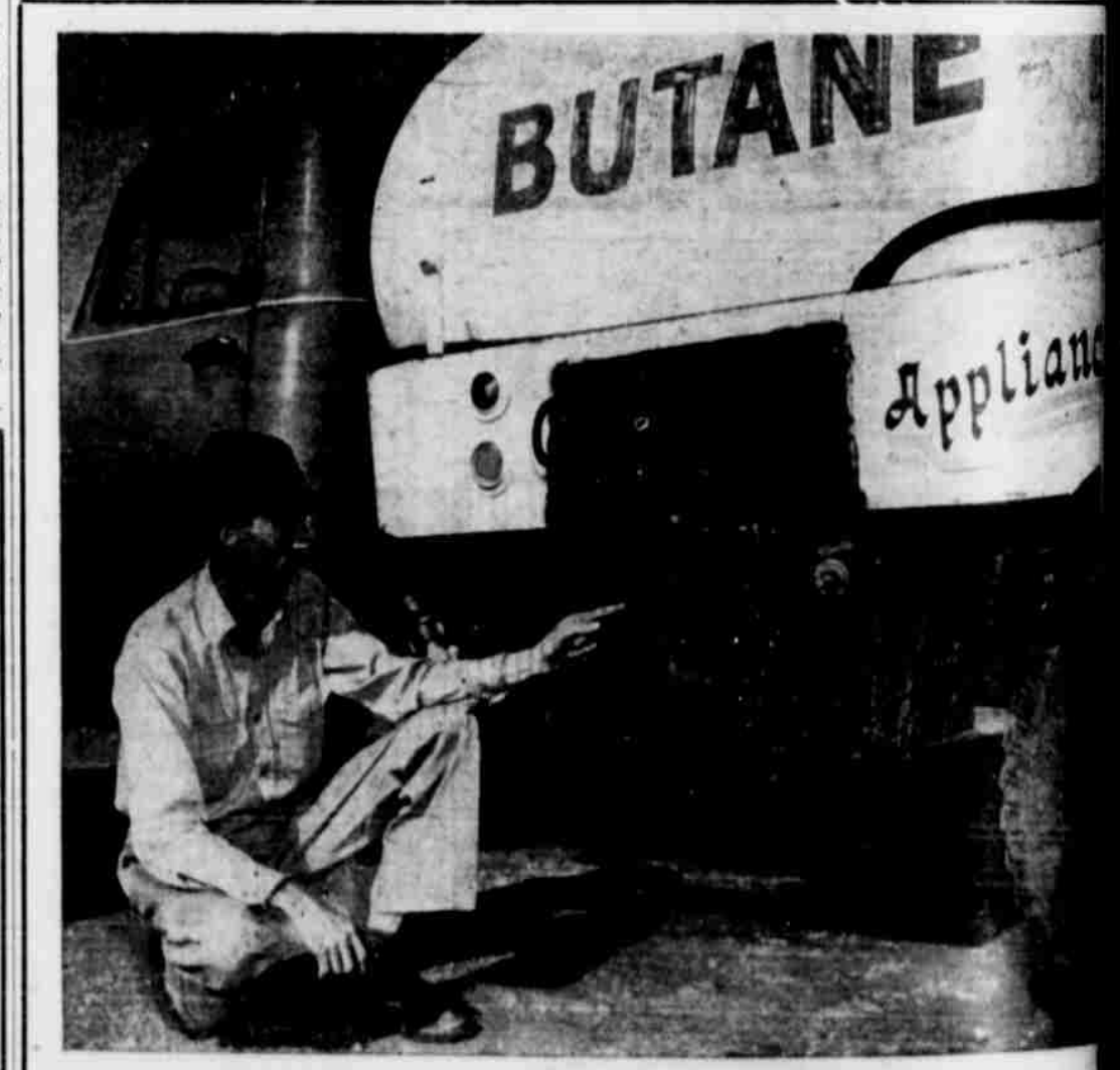
Pictured above is Thurman Maddox pointing to the new meter we have installed to give you accurate measurement on your butane orders.
