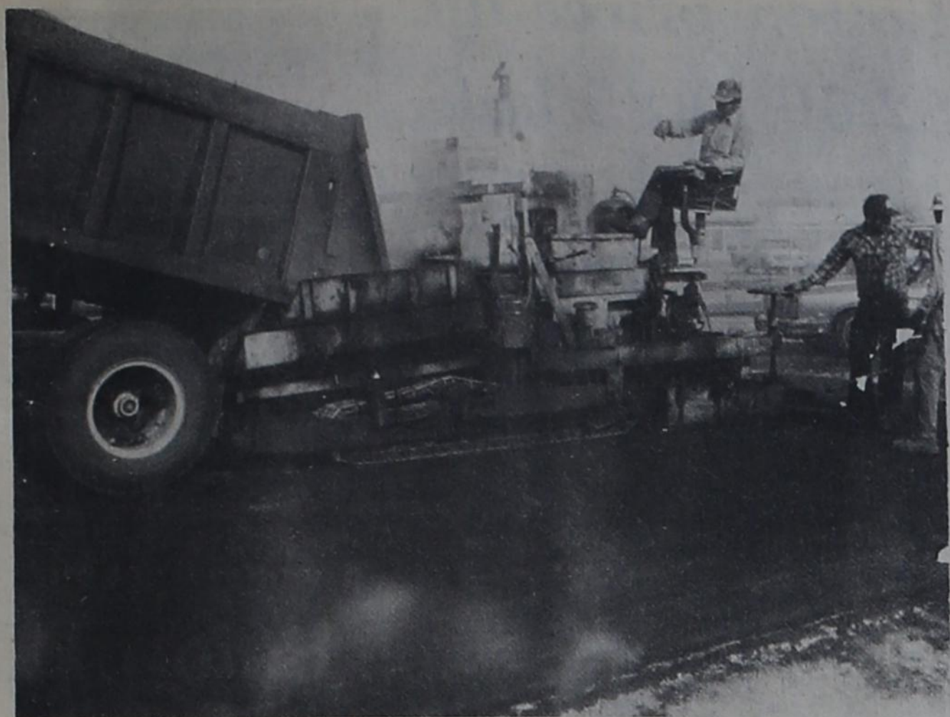
TOPPING ALL-WEATHER TRACK — Employees of Williams & Peters Dirt and Paving firm of Lubbock are shown applying the rubberized hot mix surface to Post High School's new all-weather running track Tuesday. Bad weather prevented their return Wednesday to line the new track. It will be so soft and smooth you can run on it barefooted. — (Staff Photo)
