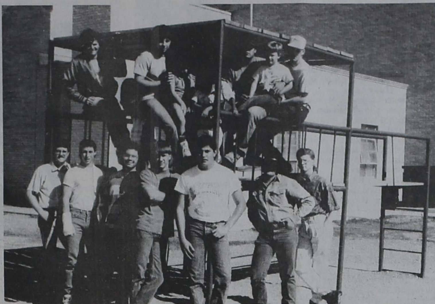
NEW PLAYGROUND EQUIPMENT - Members of the senior ag mechanics class at Post High School recently completed the construction and installation of new playground equipment for the elementary school. Participating in the project were (top row, left to right) Tracy Albert, Chris Redman, Jr Ray Gonzales, Randy McKee, (bottom, left to right) instructor Perry Smith, Scott Haynes, Benji Vargas, Dustin Massey, Joe Garcia, Jerry Hodges and Shane Johnson. Smith expressed appreciation to Mason Bros. Construction and The George R. Brown Partnership for donating materials for the project.
