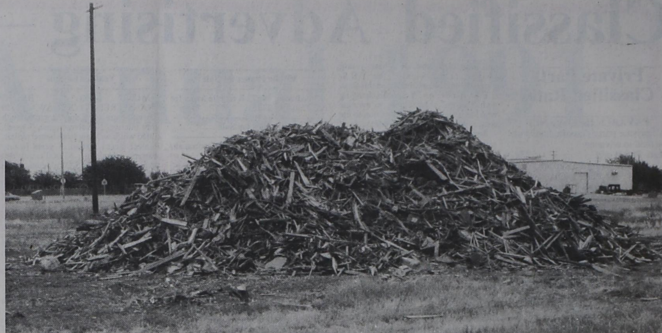
BONFIRE MATERIAL? This pile of rubbish has been stacked on a vacant lot owned by the Post ISD and was the subject of a heated debate during Monday's regular city council meeting. The debris is from the demolished old gymnasium and other materials from condemned property had been planned to be added to the pile for use in a school sponsored bonfire in September. The rubbish pile is in violation of the city ordinance pertaining to trash removal, but the ordinance was ignored by council members when discussing the issue.
