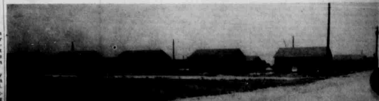
MILL HOUSES GOING UP —Shown here is the new housing addition going up in connection with Postex Cotton Mill's current expansion program. Twenty units, each with four rooms and bath, are being constructed under the mill's contract with Higginbotham-Bartlett Lumber Co. The addition is expected to be completed by around Sept. 1.—(Dispatch Staff Photo.)
