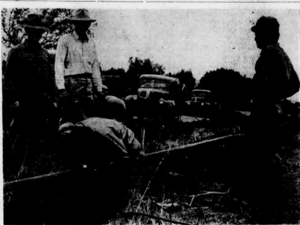
Dick Woods, left, local manager for the West Texas Gas Company and two men from the George R. Tucker Construction Company of Odessa watch Tucker Company welder work on a portion of two-inch high pressure line recently installed in north, south and west Post to accommodate 24 new consumers. Many more feet of new line will be installed here before summer is over, Woods said. This is part of the company's expansion program.
