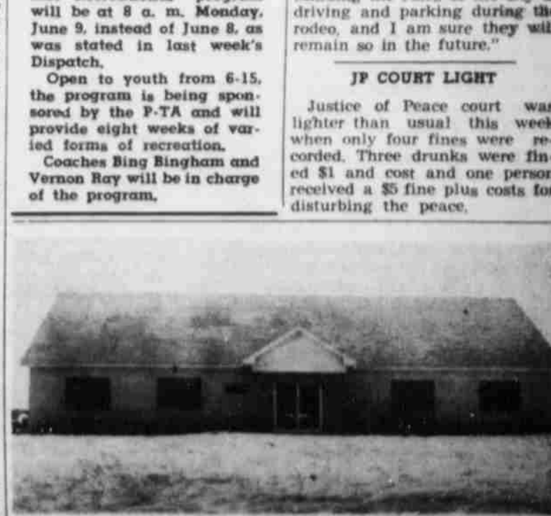
NEW SCOUT DINING HALL—Construction has recently been completed on the new dining hall donated to the South Plains Council, Boy Scouts of America, by the First National Bank of Lubbock. The new structure, located at Camp Post, 2 1/2 miles southwest of Post, will seat approximately 400 persons. See story of Scouting on inside page.—(Dispatch Photo).
