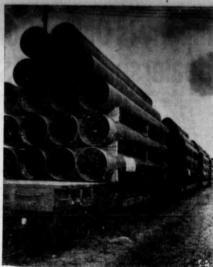
MILES OF PIPE —These sections of pipe for the construction of another "big inch" pipeline for the Tennessee Gas Transmission company were unloaded at Banquete, for the second section for a 2,000 mile gas line that will terminate in New York. A total of 150 carloads of pipe, 17 to a car, have been stockpiled for the 70-mile section between Agua Dulce and Edna, in South Texas.
