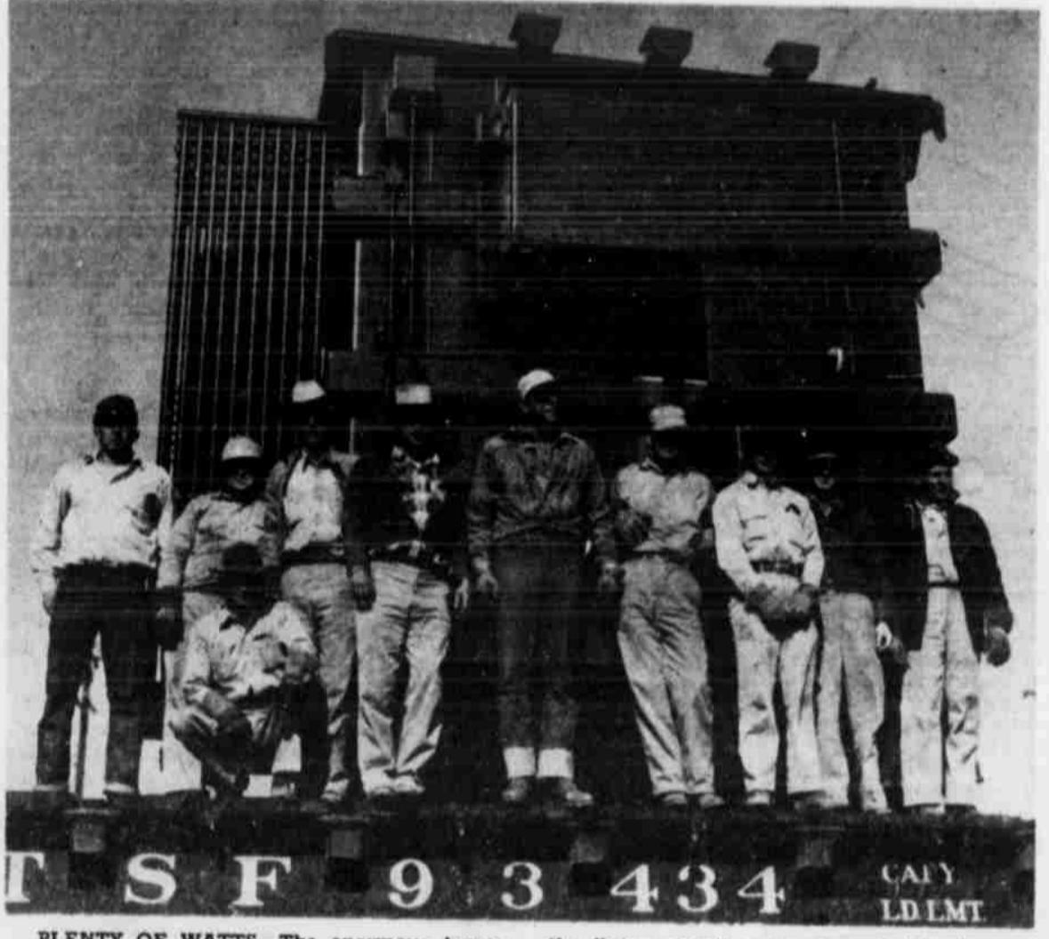
PLENTY OF WATTS—The enormous transformer pictured above will carry plenty of electric power to Post residents in the next year. Being installed to replace an older and smaller unit, the unit is pictured while still on the flatcar at the railroad yard. Its size can be compared by the way it towers over the crew which unloaded it for Southwestern Public Service. (Photo by Dispatch Photographer.)
