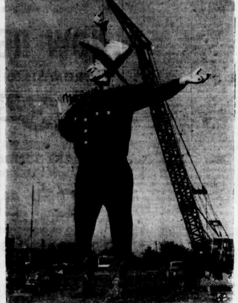
TEX COMES DOWN—Tex, the 52-foot-high cowboy figure which stood at the State Fair of Texas in Dallas, begins coming apart at the neck as workmen dismantle him for storage. Riding on the line above the hat is Jack Bridges, the artist who designed the figure of steel, papier-mache and cloth. Bridges had a half dozen helpers and 25-ton crane to take Tex apart.
