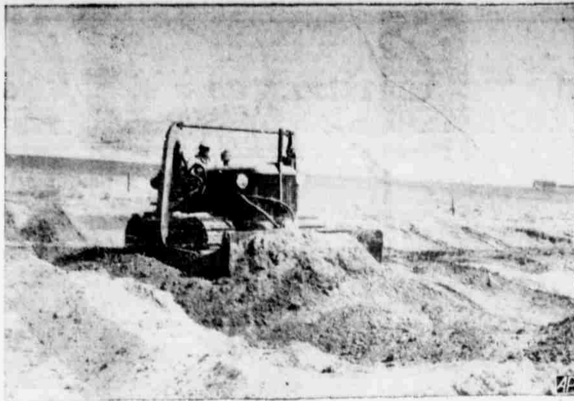
THERE'S A RAILROAD UNDERNEATH —Dust storms, which whipped across the South Plains of Texas buried two short sections of Santa Fe Railroad tracks west of Brownfield, Tex., and bulldozers were called in to move the main portion of the sand so that work gangs could get to work to clear the rest of the track bed. At this point, the sand was as much as two feet deep over the rails.
