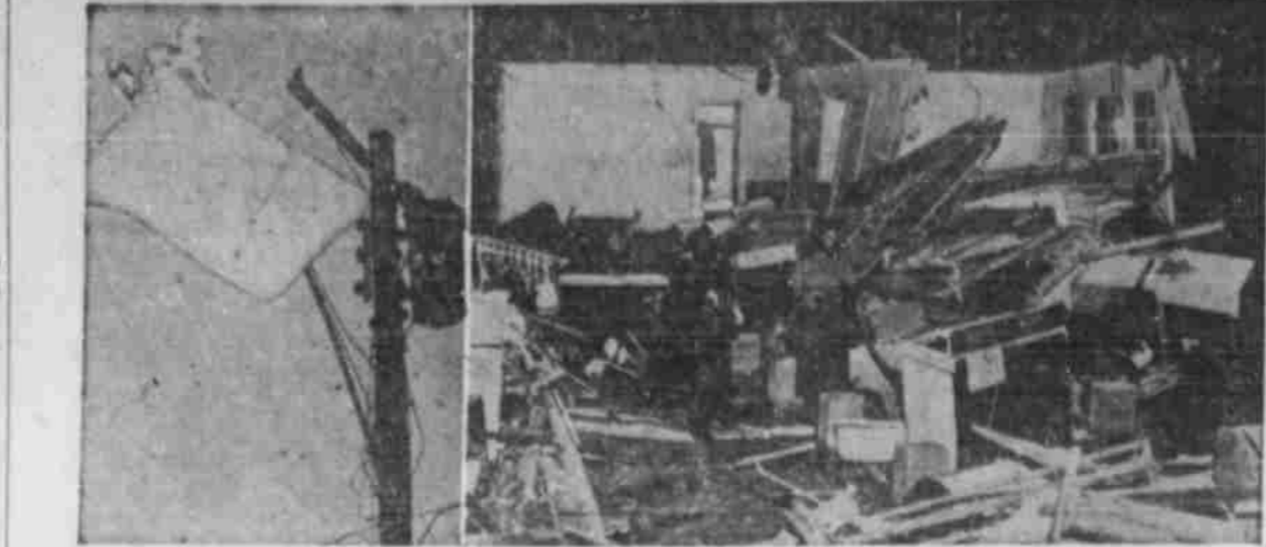
TORNADO TERROR was visited on this west Dallas apartment house (right), while the twister which hit the afternoon of April 2 also showed a grisly pranksiness (left). Returning residents found only debris, and workers from Dallas County Civil Defense, police, firemen and Red Cross guarding the wreckage and ready to provide temporary shelter. (Dallas Morning News Photos)
