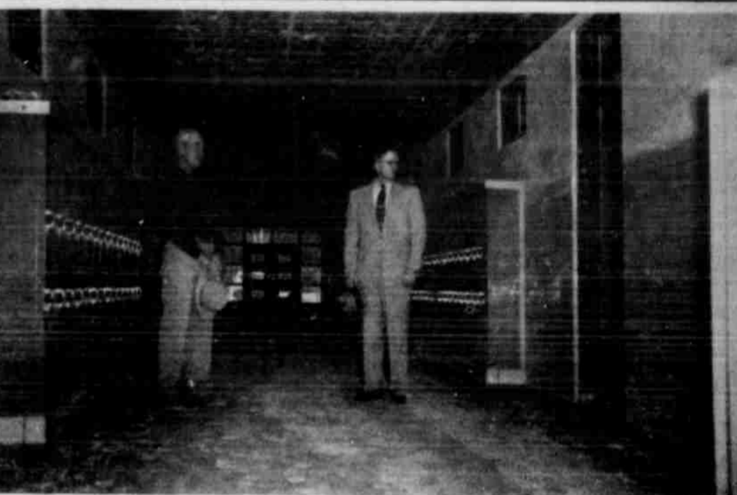
LOOKING OVER NEW SCHOOL — Tom L. Sampson, contractor (left), and Ellis M. Mills, grade school principal, are shown in the corridor at the new junior high school building nearing completion here. Far down the corridor is the west entrance to the front part of the building.—(Staff Photo).
