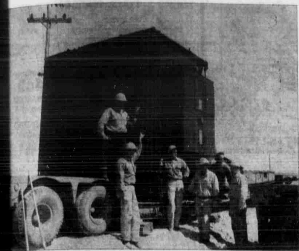
35-TON UNLOADING JOB FOR SWPS
