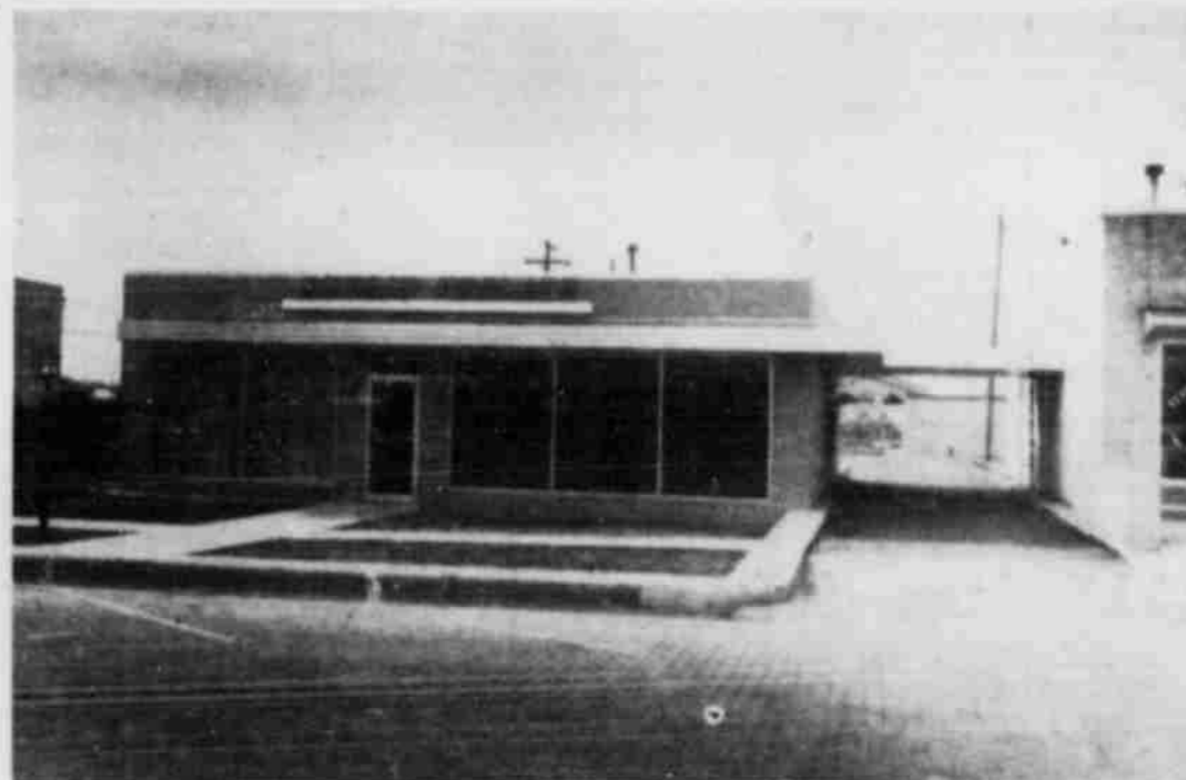
NEW PUBLIC SERVICE OFFICE AT 217 WEST MAIN STREET
