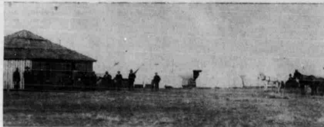
COMMISSARY, HEADQUARTERS BUILDING
