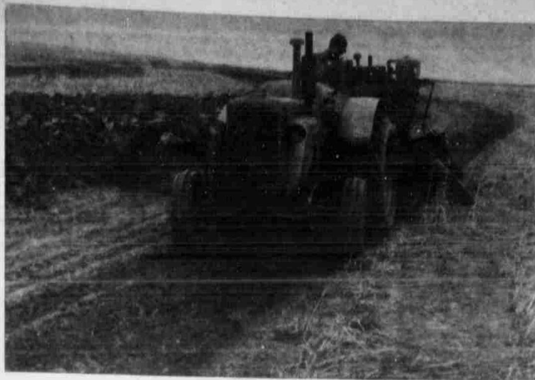
WORKING ON FARM TERRACES
