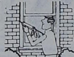
Caulk around doors and windows
