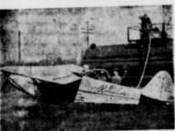
For the first time, liquid nitrogen fertilizer was transferred direct from a railroad tank car to a waiting plane. The plane flew 20 miles to a 1000-acre wheat field, sprayed its load, and returned to the siding for a quick refill-all in about 15 min-
