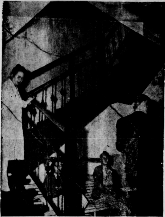
IRON STAIRS IN ABILENE HOSPITAL — This ancient iron stairway at the Abilene State Hospital has caused many falls—not only by the epileptic patients in the hospital, but by the nurses as well. Several patients in the last dozen years have fallen on these stairs and been killed. Injuries occur nearly every week. Notice how cautiously the nurse in the picture is moving from step to step. Abilene State Hospital was one of the several hospitals at which newspapermen of the state recently inspected conditions.
