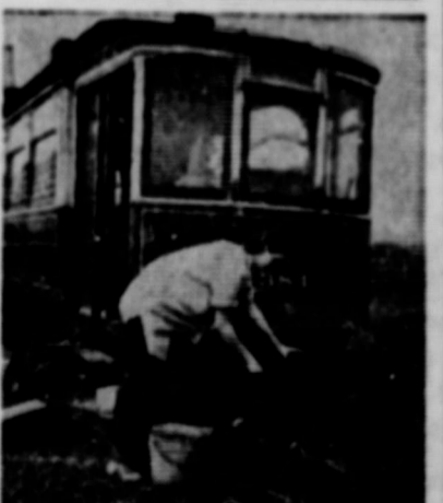
With typical American ingenuity, the Sands of Chicago, Ill., solved housing shortage by buying old street car for $200 and converting it into dwelling. This is one of several hundred old trolley cars which were sold by a street railway company to veterans rather than burn them as is usually done.
