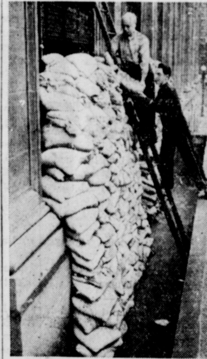
Completing the job of placing sandbags outside the office windows of Hotel Bossert in Brooklyn. The barriers were installed so the hotel organization could keep functioning in case of an air raid.
