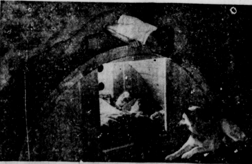
If the brick of this house comes tumbling down, the mother and two children inside this timber air raid shelter would be fairly safe. The heavy timber is easily put together with pegs, contains a double bed and incendiary bomb fighting equipment. The family is bundled in for the night, with one son on top, looking on—and the dog looking in.
