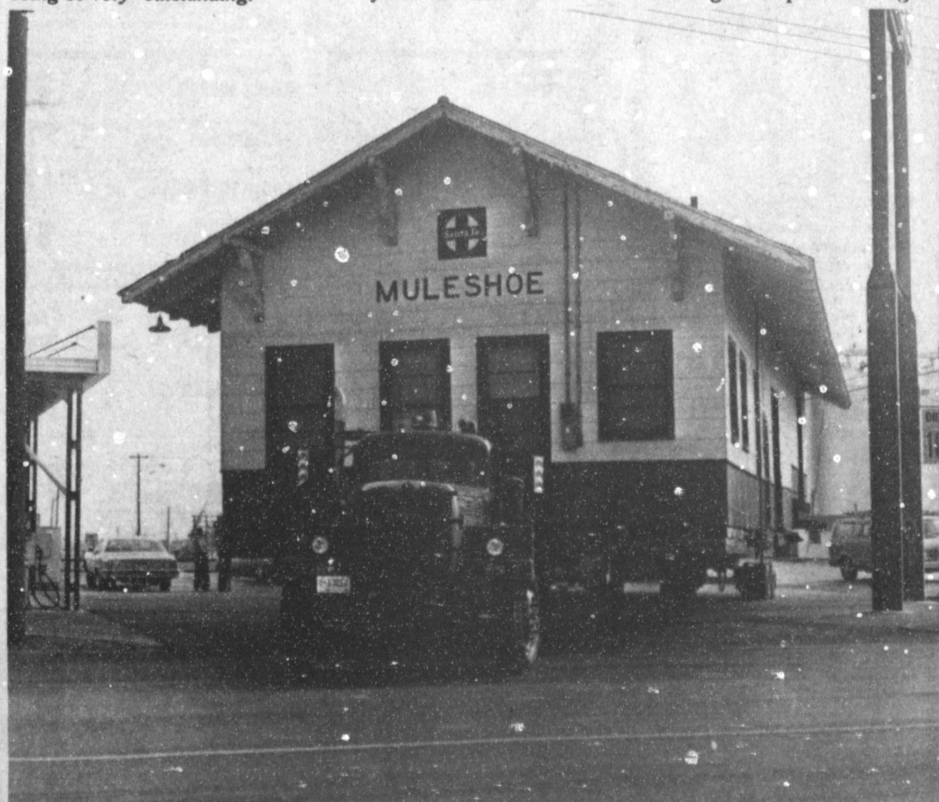
MULESHOE LANDMARK MOVED FRIDAY--On the way to a new historical complex located to the east of the Mule Putt Miniature Golf Course, the Santa Fe Railway depot, which stood at the north end of Main Street for more than 60 years, will become a senior citizen's center and a museum. Under auspices of the Bailey County Historical Commission, the depot is the first of three historical buildings to be moved to the new location. Renovation is expected to get underway in the near future.
