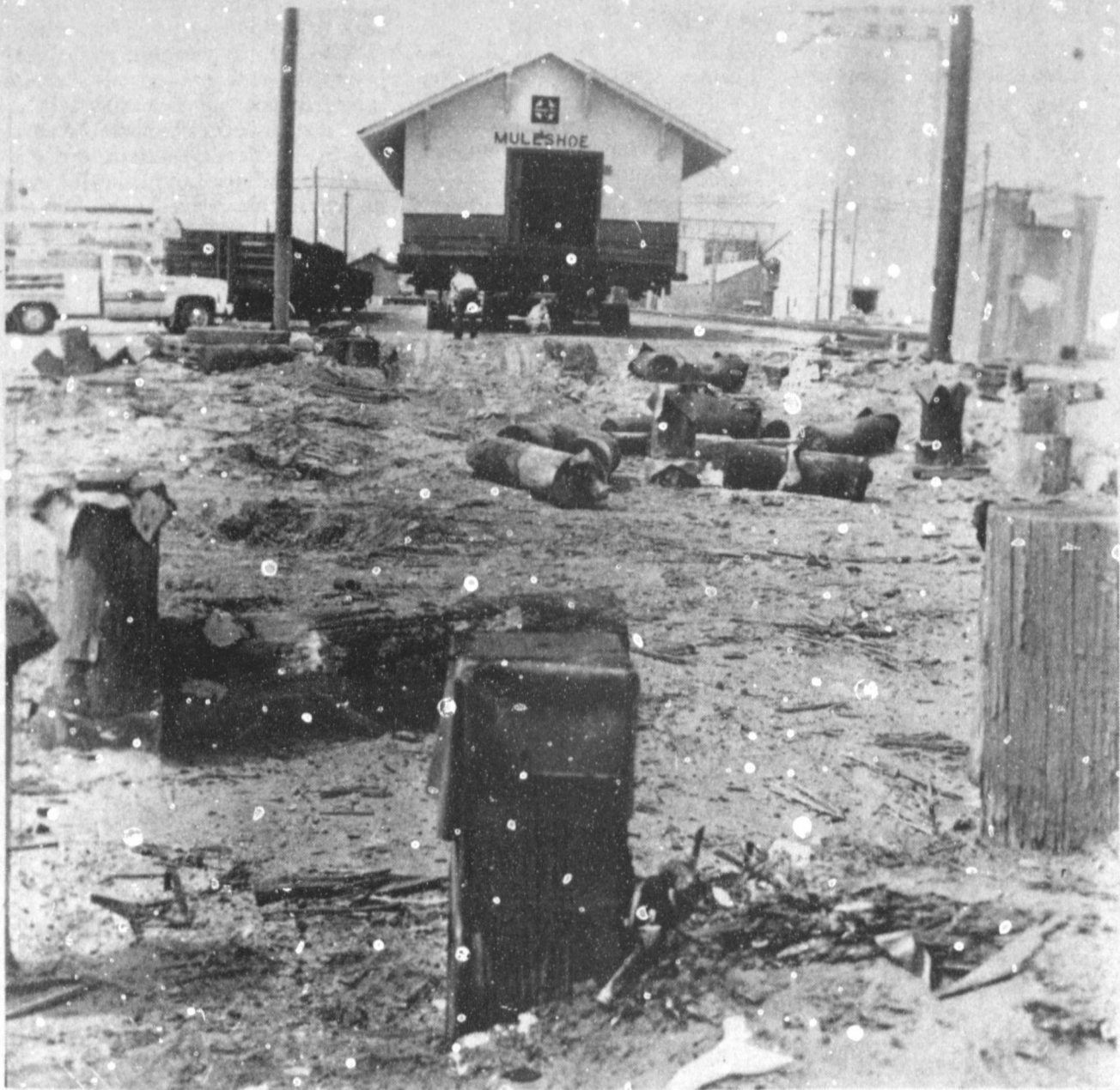
DEPOT PREPARED TO MOVE --Monday, shortly after lunch, this was the scene as the former Santa Fe depot was jacked up and moved off its foundation, in the foreground, in preparation to move it to location east of the Mule Putt Miniature Golf Course. Privett Movers had the old landmark ready to start moving shortly before 9 a.m. on Friday, as SPS employees, along with workers from General Telephone prepared to move lines out of the way.
