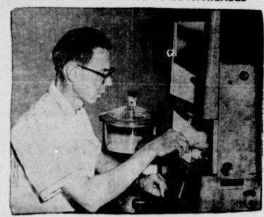
Area Soil Chemist James H. Valentine, A. and M. College Extension Service, has completed preparations for the formal opening of a new Soil Testing Laboratory in Lubbock. Abive, he is making a final check of the delicate chain balance which is used to measure the minute quantities of chemicals required in running a soil analysis.
