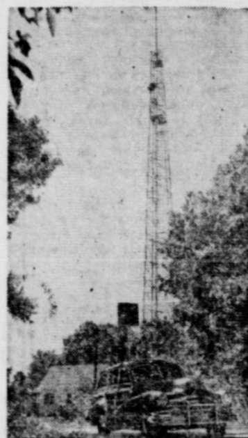
SUCCESS HILL —The lofty antenna of the Bridgeport UHF station towers over the white frame station house at the left. In the foreground is a station wagon equipped with UHF receiver and portable antenna. It has been used to test signal strength throughout the Bridgeport area. Station KC2XAK is the first and only UHF station in the country to operate on a regular daily basis. It is located on the crest of Success Hill on Bridgeport's outskirts.
