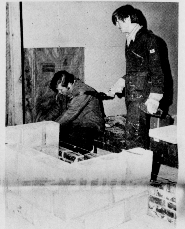
MASONRY WORK includes fireplace.
