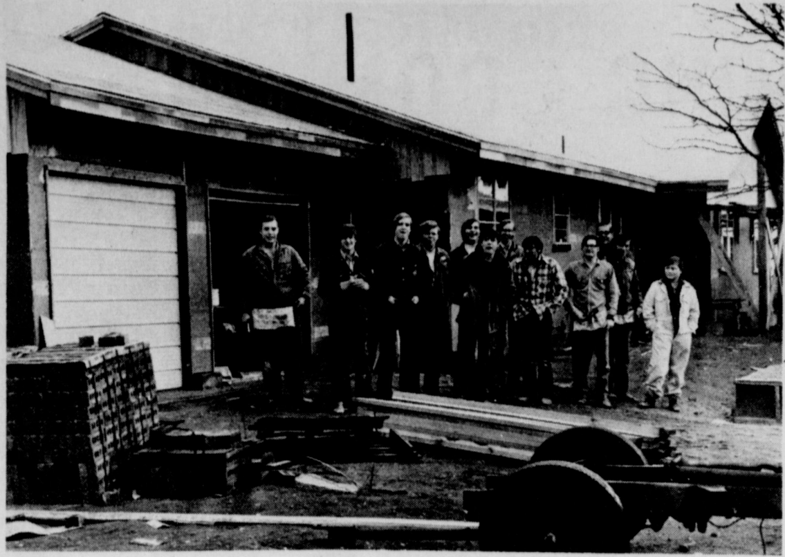
STUDENT-BUILT HOME is fronted by members of the morning Building Trade class.
