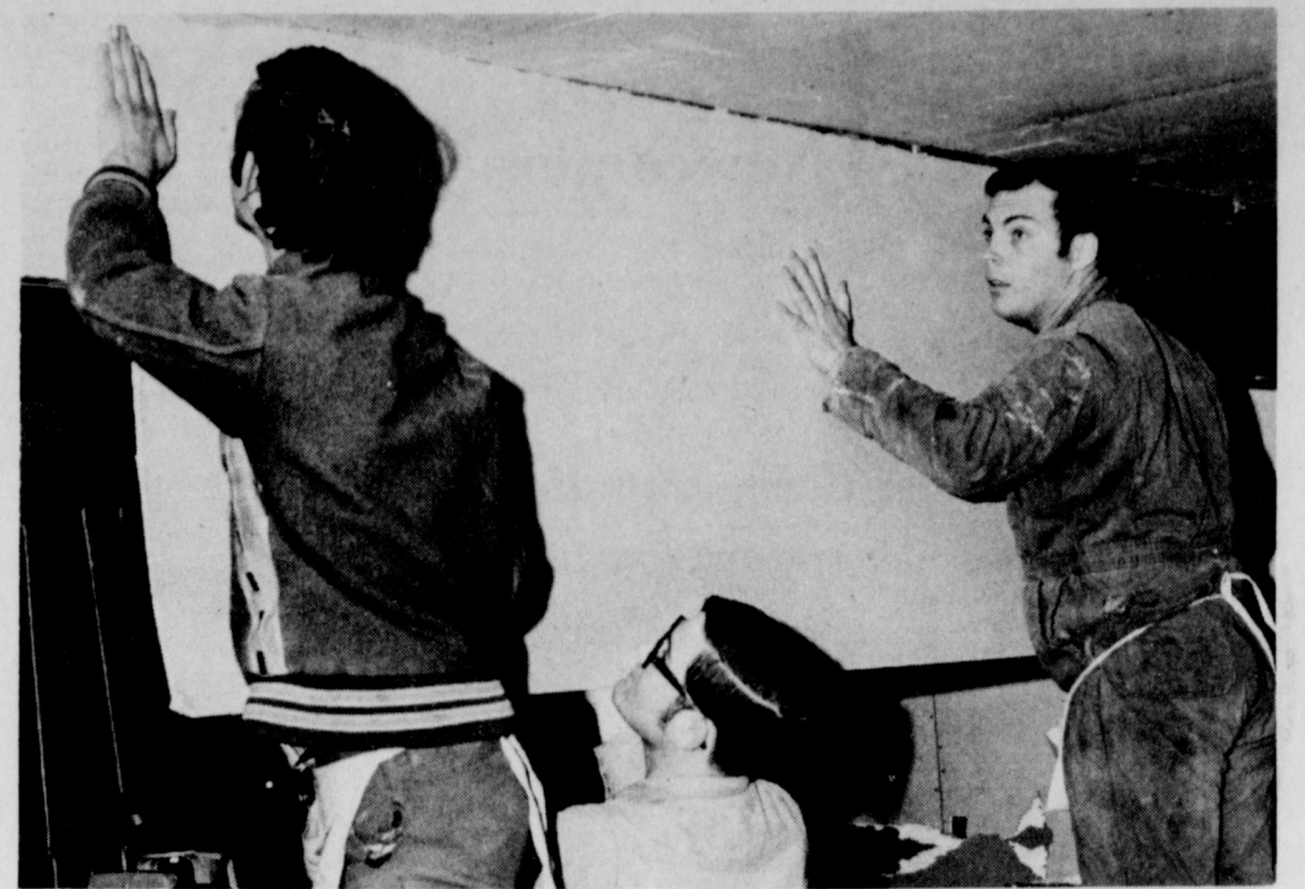
SHEET ROCK for walls going into place.
