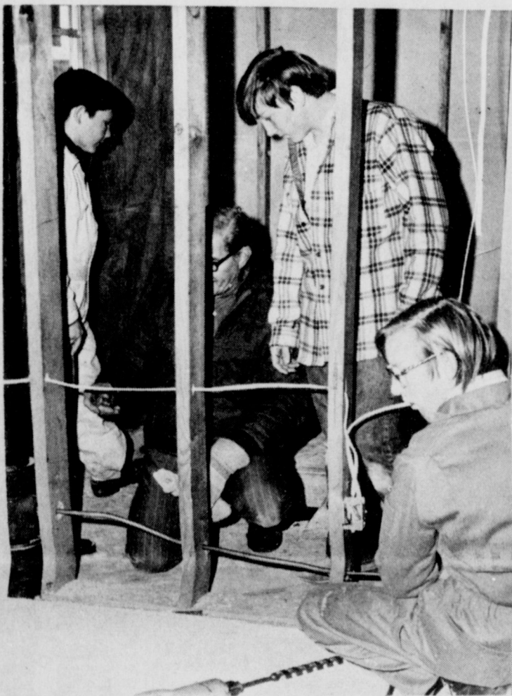
COPPER TUBING for plumbing nearing completion.
