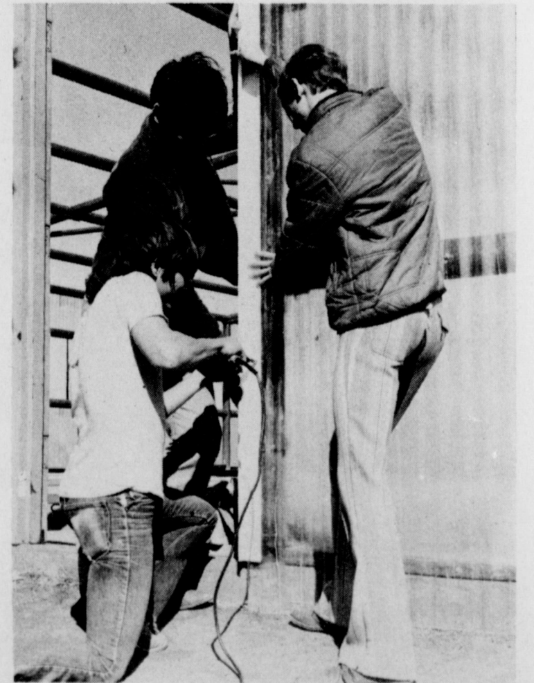
NEW GREENHOUSE is being built by students themselves.
