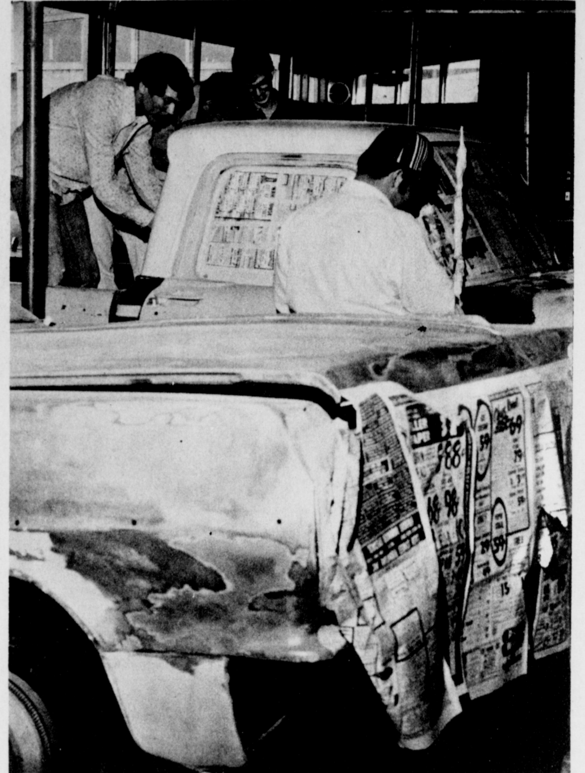
BODY REPAIRS include painting, and that takes big masking job.
