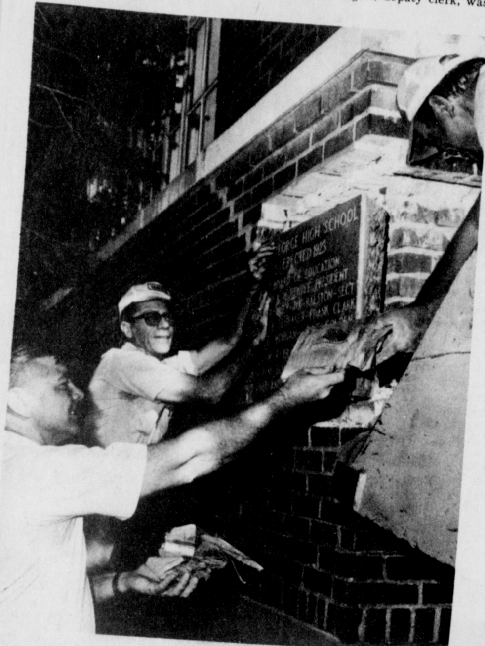
CORNERSTONE TREASURE - When the W.F. George school building's cornerstone was opened Wednesday morning, evidence of the past was recovered. Kenneth Watts, of the maintenance department, pulls the papers out for Harold Cowley, representing the school, while Jesse McCullough, representing the Masonic Lodge, looks on.
