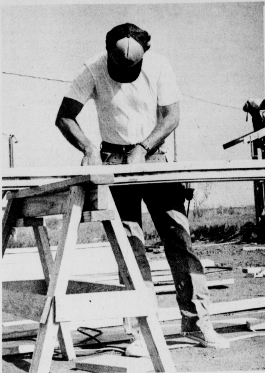
CONSTRUCTION OF NEW HOMES UNDERWAY ... prospective growth in Holliday being realized.
