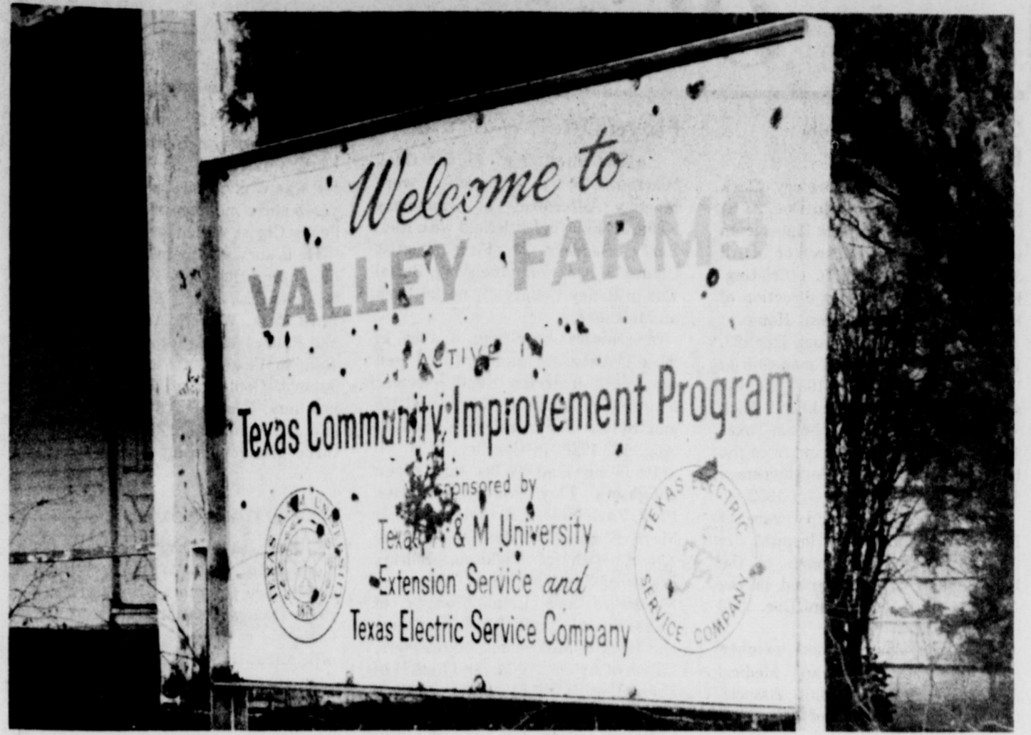
SIGN IN FRONT OF VALLEY FARMS COMMUNITY HOUSE . . . in better condition than building itself.
