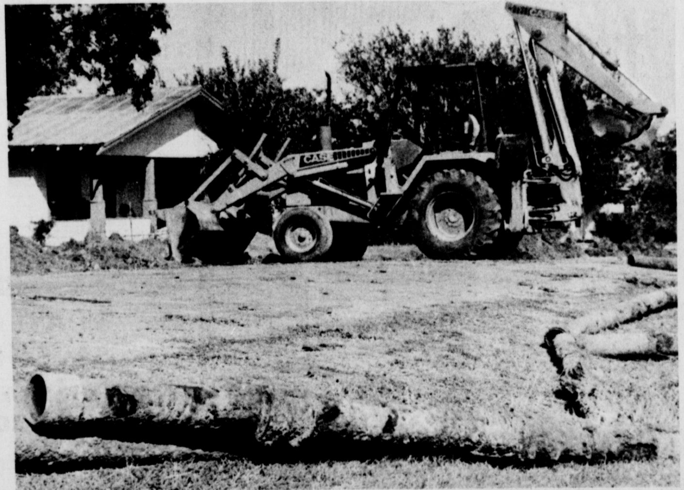
WATER LINE REPLACED - City workers early this week replaced the water line of 400 East Bank. Date of installation of the steel pipe is unknown, but like other
