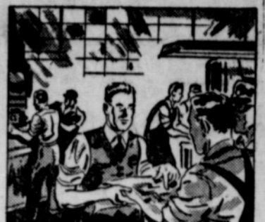
2. THURSDAY NIGHT: As many workers as could be efficiently employed on the job worked all night, all day FRIDAY, assembling the equipment.
