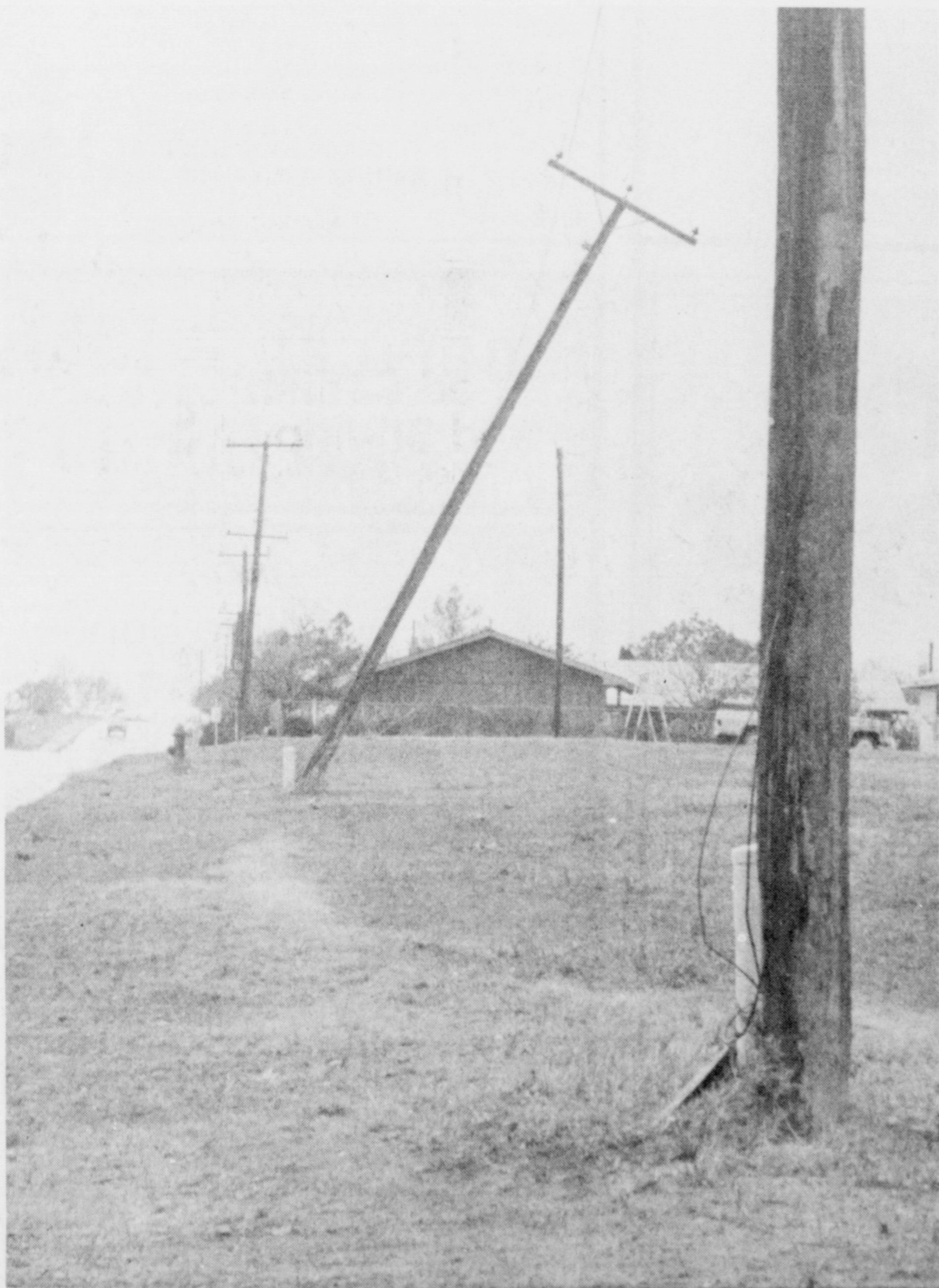
BROKEN HIGHLINE POLE ON THIRD STREET
