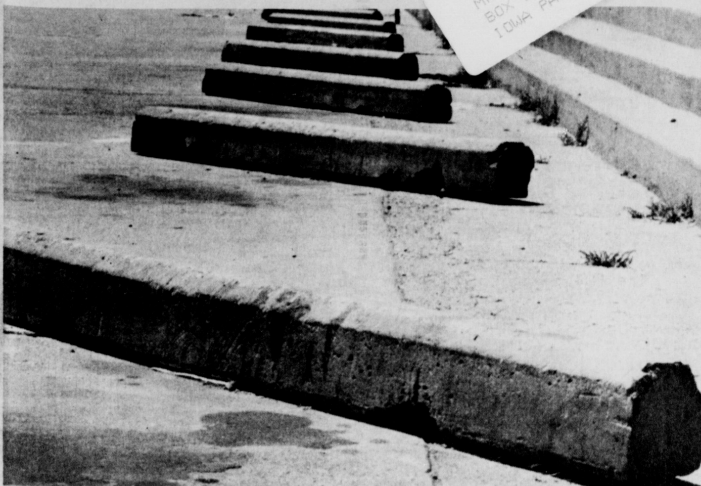
ABOUT TO DISAPPEAR - The familiar concrete parking blocks on West Cash will be gone in about a month. City council members gave the thumbs down on the blocks last week, on the basis so many vehicles had sustained damage from them, primarily the stakes that are supposed to keep the blocks in place. Parking lanes will be painted and supplemented by reflector discs.
