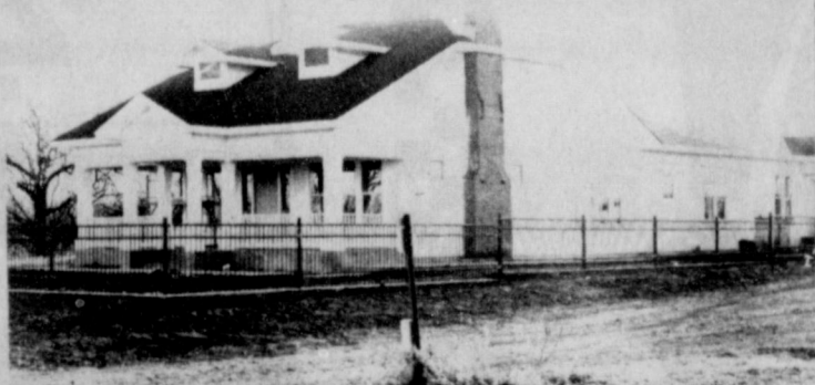
After - Job Completed by Johnson Siding
