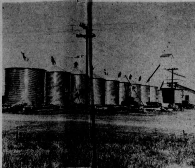
The wheat storage facilities of this farming area were greatly augmented this year when L. I. Southard built nine new all metal bins in connection with his elevator business in Iowa Park. They are situated along the Fort Worth & Denver railway tracks and give the town a trim and prosperous look. The main elevator is at right.
