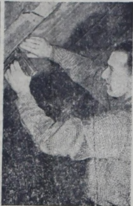
Stapling mineral wool blankets is generally faster and more efficient than nailing.
